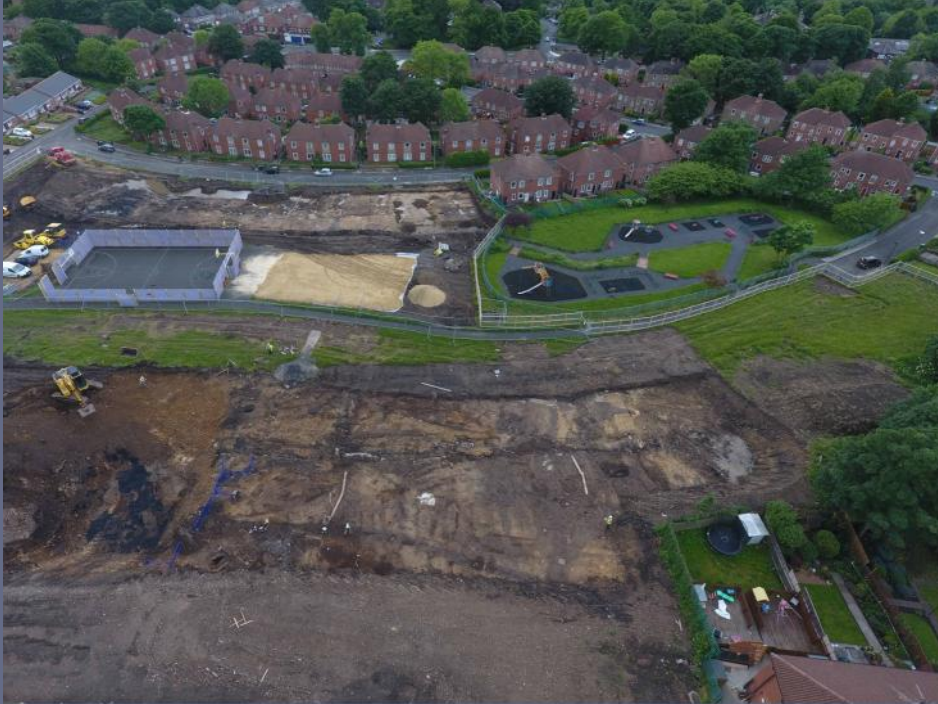
Aerial view looking south, showing the north and south excavation areas
